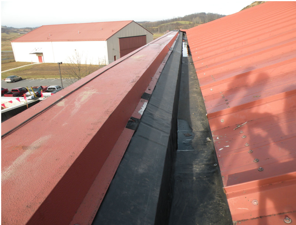
2014 Post Gutter Repair
