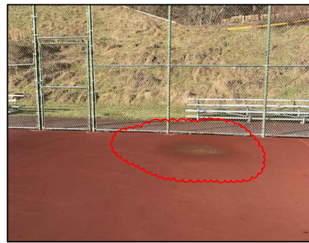
#5 Repair low spots- bird bath.. Patch w/ Latex-Ite Acrylic Patching & Leveling Compound
